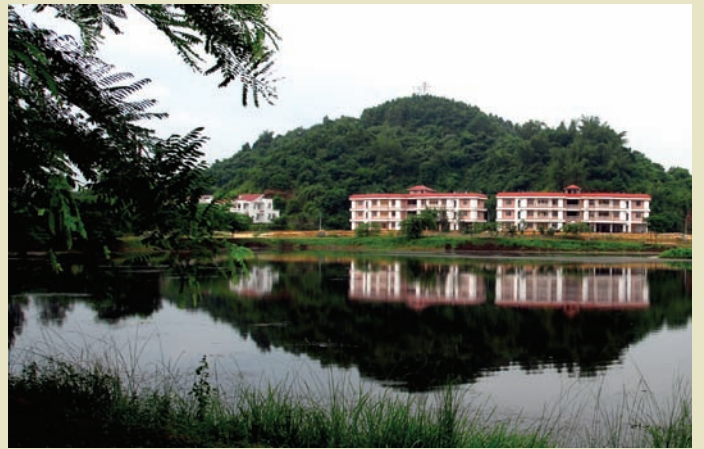
Newly completed faculty quarters by the serpentine lake
